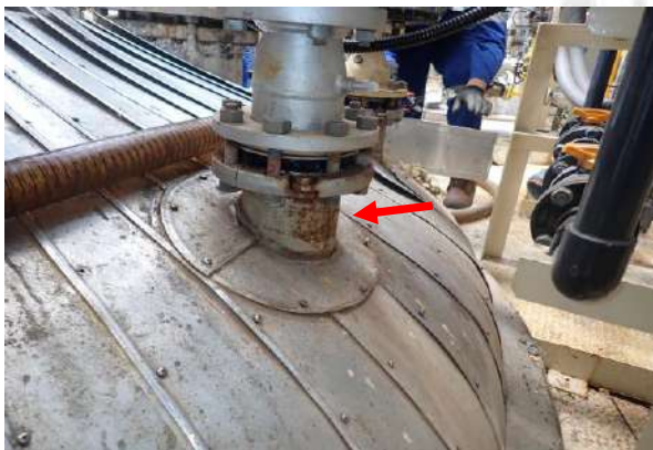
Found rust on nozzle and flange.
