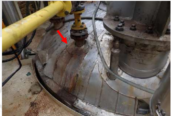
Found damage on insulation cover.
