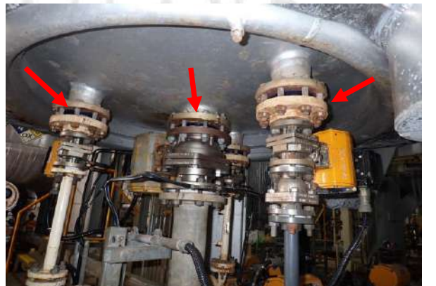
Found rust on flange of bottom head.
