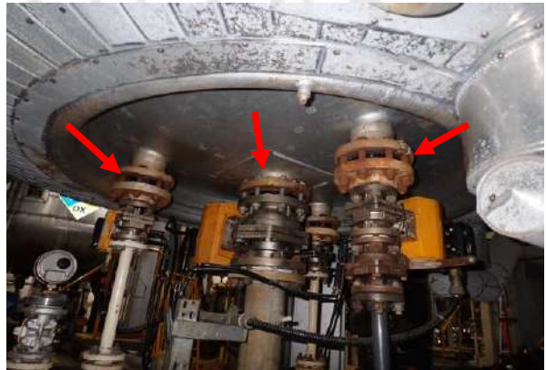
Found rust on flange of bottom head.
