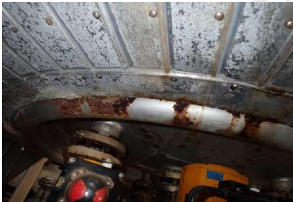
Found moderate corrosion on bottom head.
