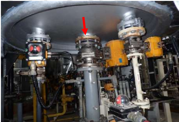
Found rust on flange of bottom head.
