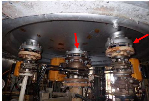
Found rust on flange of bottom head.
