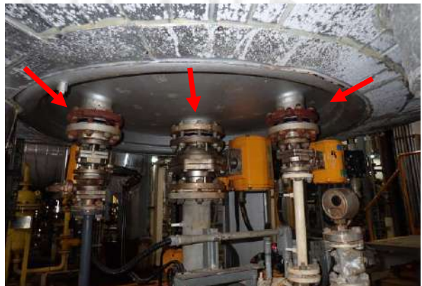
Found rust on flange of bottom head.
