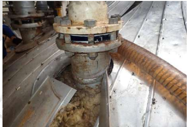
Found rust on nozzle and flange.
