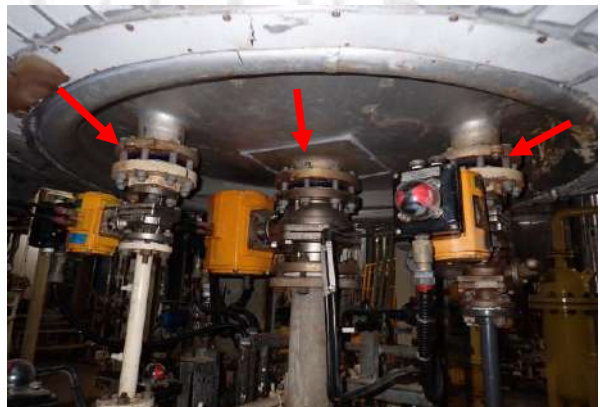
Found rust on flange of bottom head.
