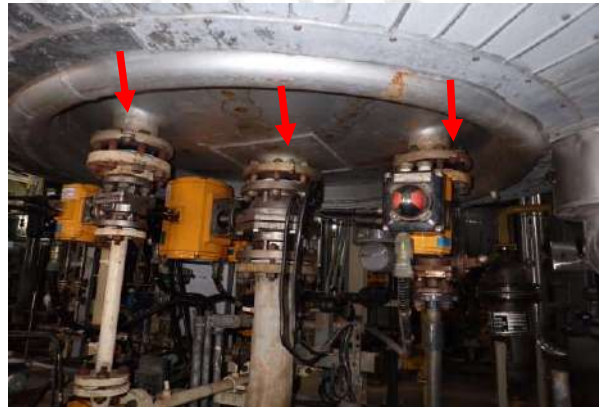
Found rust on flange of bottom head.
